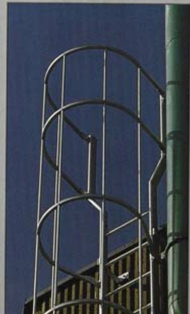
EXTENSION ROOF ACCESS
