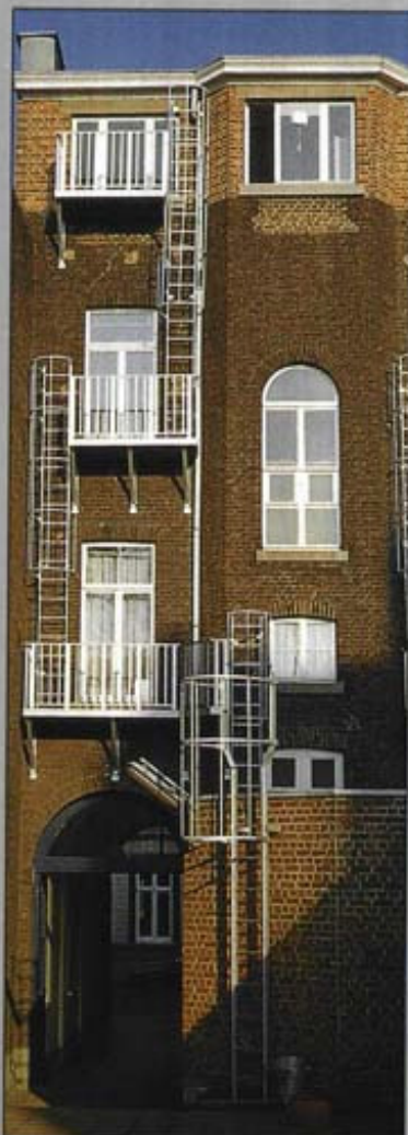
ACCESS BALCONY ON REAR OF BUILDING
